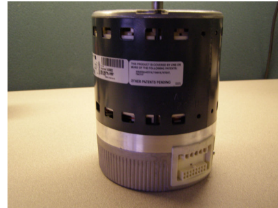
Figure 7: Motor and control mated
